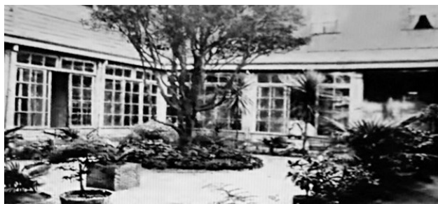
Patio interior Concepcion College .
